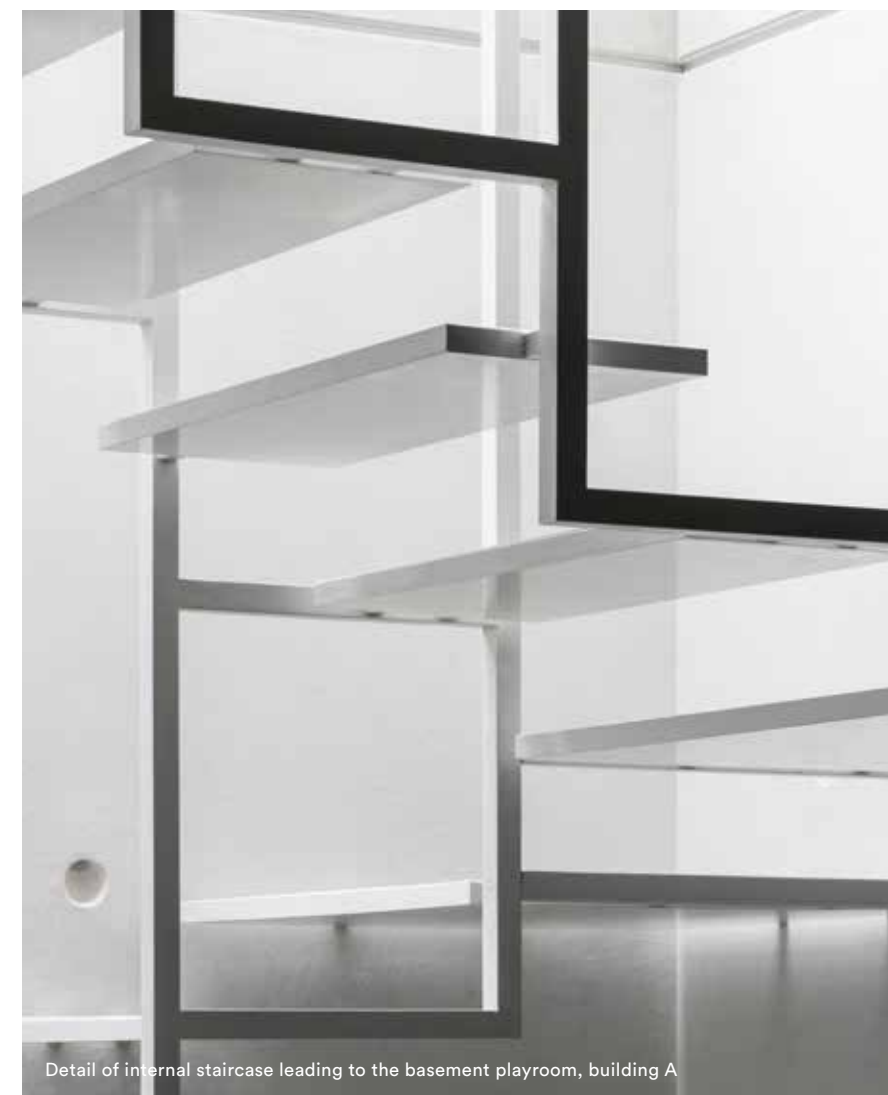
Internal white metal staircase leading to basement playroom, building A
